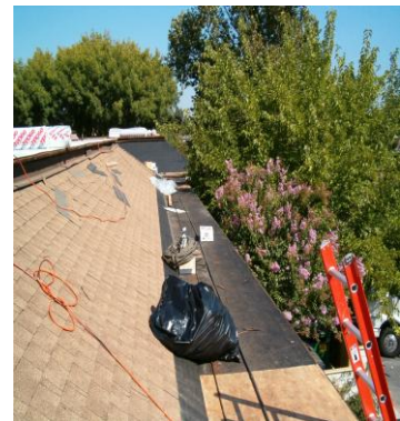
New Sheathing & Shake
